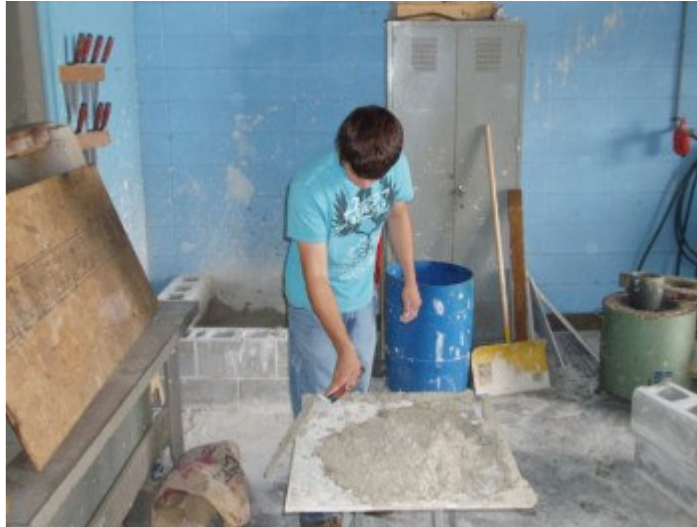
Cord Anderson practicing the correct trowel holding techniques along with spreading mortar down the edges of his mortar board.
